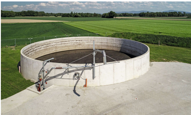
Fig. 5: Ready-mixed concrete containers
