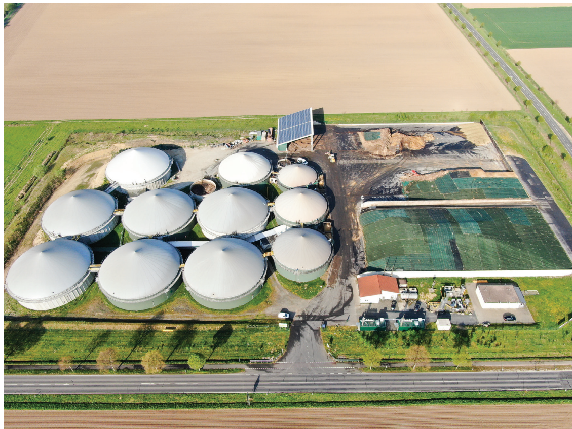
📍 Fig. 3: Rosdorf biogas plant
