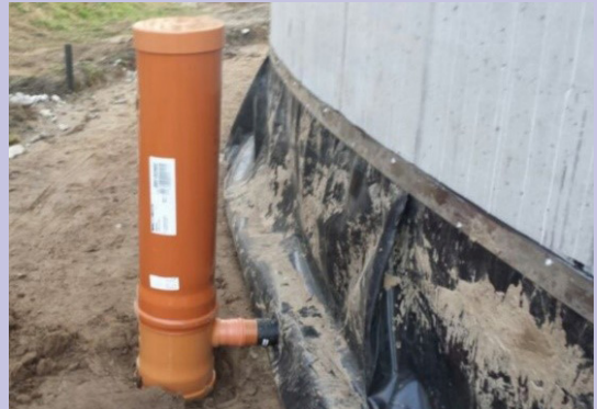
Fig. 9: Drainage pipe with inspection tunnel
